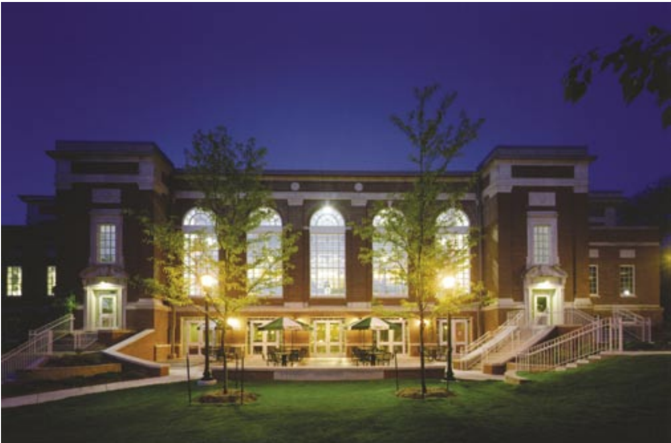
(Title page) Existing Memorial Gymnasium offered the perfect site for the new Student Center. The exterior was rehabilitated to honor the building's historic significance, as well as its important new function. (Above) At night, the Hansen Center glows like a beacon, welcoming the University community to this important campus precinct.
